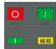
Circuit breaker closed and energy storage completed state
