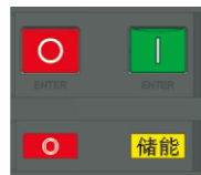
The circuit breaker is off and the energy storage is complete
