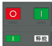
Circuit breaker closed and no energy storage state
