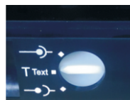
In the "test" position, the main circuit is disconnected, Secondary loop on
