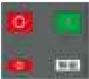
The circuit breaker is off and has no energy storage
